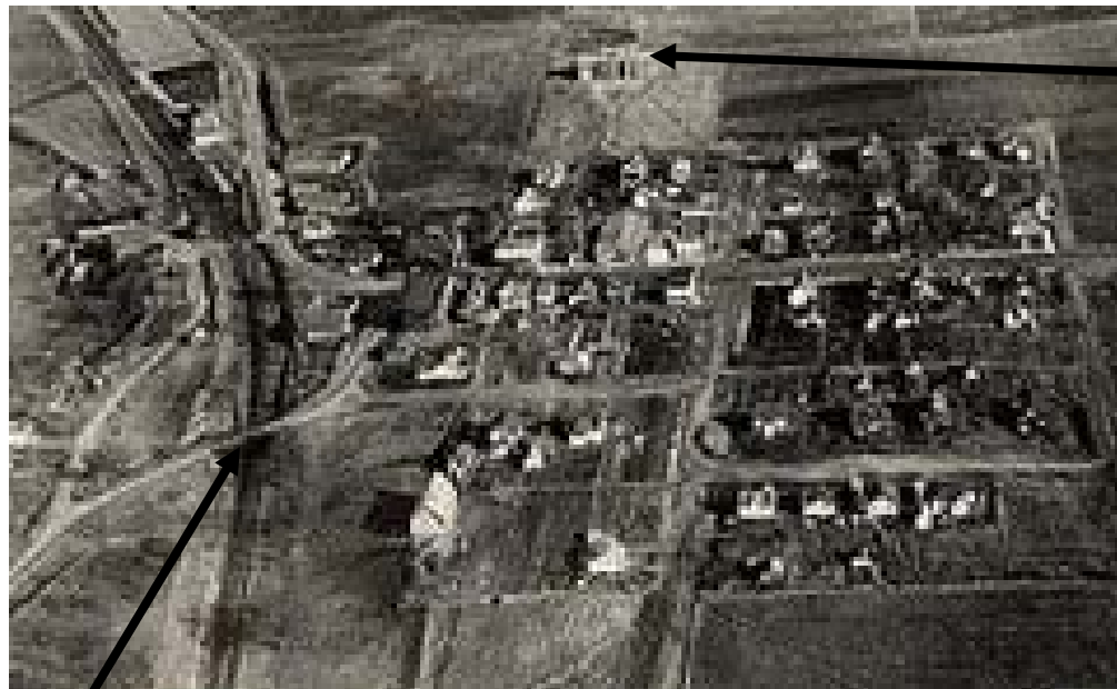
Stieger Lake Lane bridge
